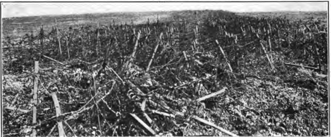
WIRE ENTANGLEMENTS IN FRONT OF HINDENBURG LINE
